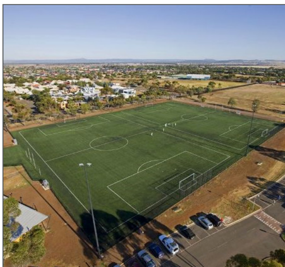
Rolls of turf installed in the same direction
