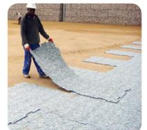
Optional Patented System: drainage cell layer under shock pad & synthetic turf eliminates all infrastructure required in base construction
