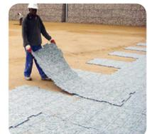
Optional Patented System: drainage cell layer under shock pad & synthetic turf eliminates all infrastructure required in base construction
